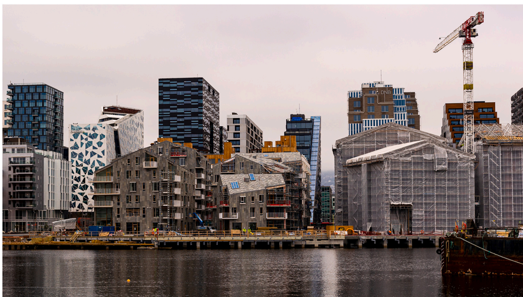
Fig. 5. The B6A/B6B (Vannkunsten) housing, building Step 1 and 2. Photo by Aleksander Bern.
