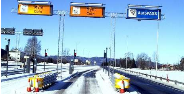
Figure 2.5: With AutoPASS you can pass the toll collection even at high speeds.
