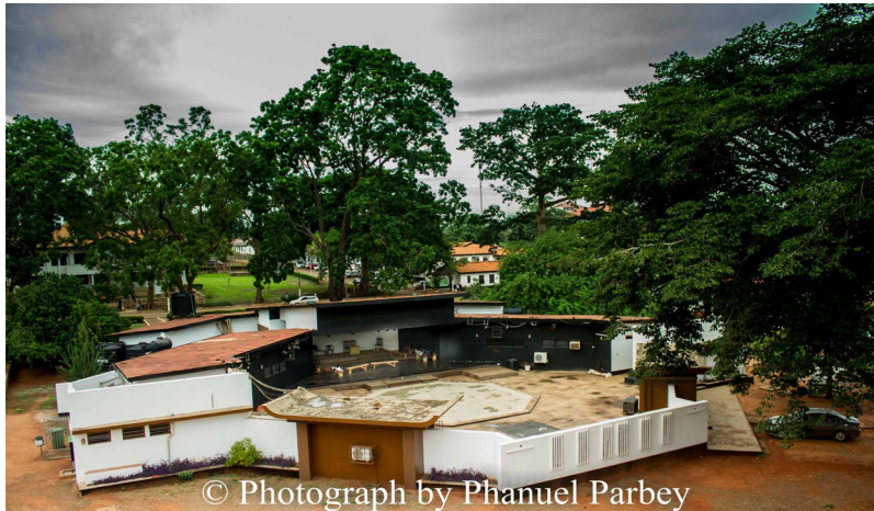
Figure 1. (Aerial view): The Drama Studio (now known as the Efua Sutherland Drama Studio) replicated and relocated to the School of Performing Arts premises at the University of Ghana. Photo credit: Phaniel Parbey.
