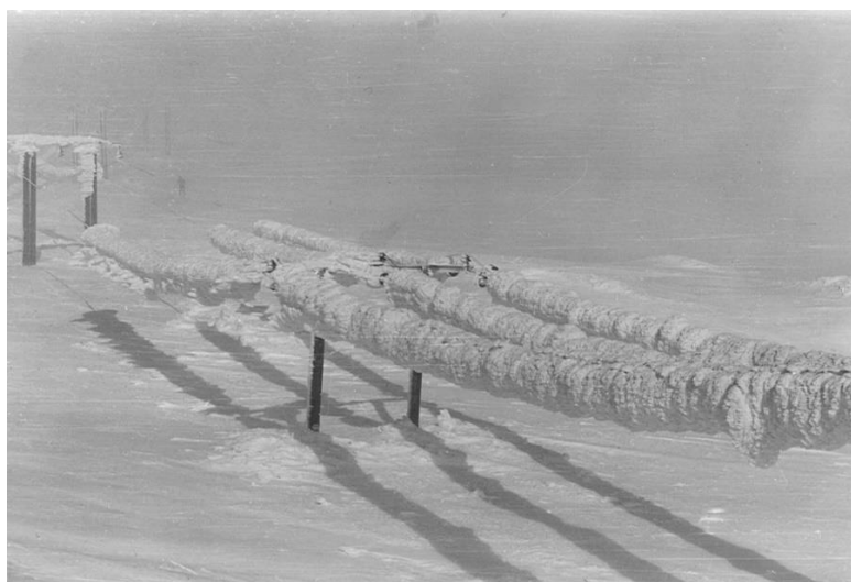
Figure 2.5: Rime ice on a power line, 1410 m.a.s.l. at Voss, Norway, in April 1961. (Photo: Olav Wist. Rights: Kjeller Vindteknikk).
