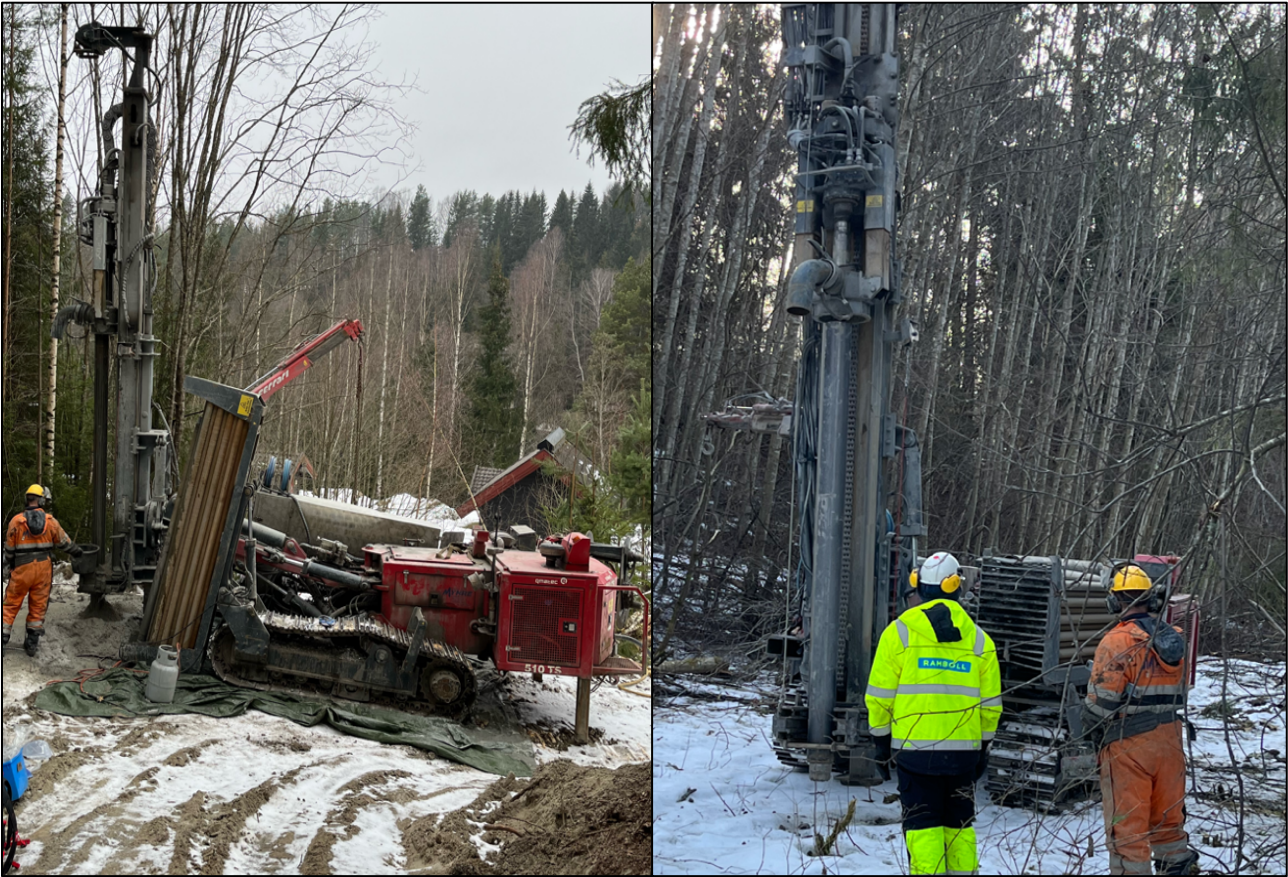
Figure 3.4. The drilling rig with odex crown showing the establishment of one of the observation wells.
