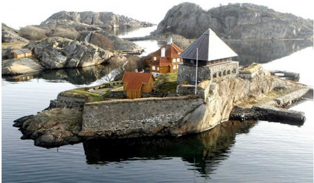
Figur 50: Stavern fort. Citadelloya, ca.1685
