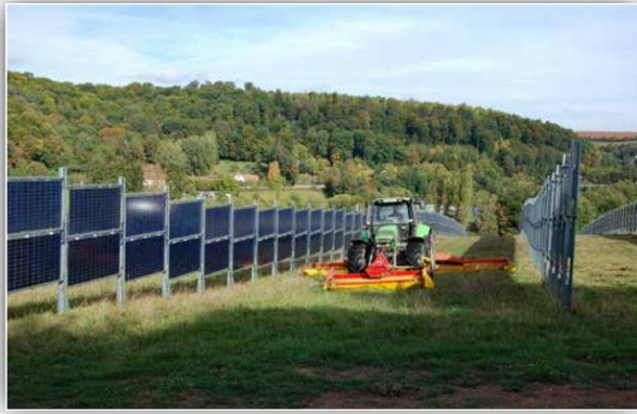
Figure 1- Vertical bifacial modules found at Eppelborn-Dirmingen solar park, Saarlans [6]
