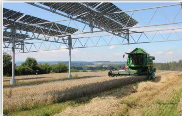
Figure 2 – vaulted PV modules with combiner underneath [6]
