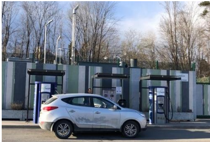
Fig. 1: Picture of a hydrogen-powered car at Høvik hydrogen fueling station in Norway (pictured 09.04.2022, established in 2019)
