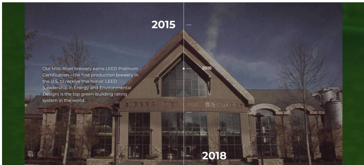
Figure 9: The Mills River Brewery. Retrieved January 11, 2022 ( https://sierranevada.com/about/our-story/ )
