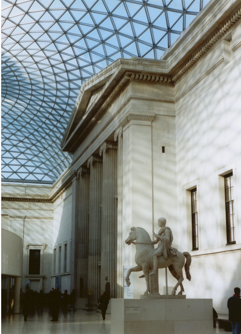
Figure 1.1: Queen Elizabeth II Great Court with a roof made with the use of generative design [15]
