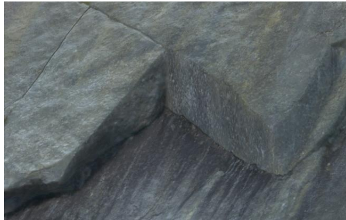
Figure 5.21 Example of a common joint configuration in Valle study area, shown on the 3D mesh model. The joints define a block with a slope parallel basal plane and wedge-shaped sides.
