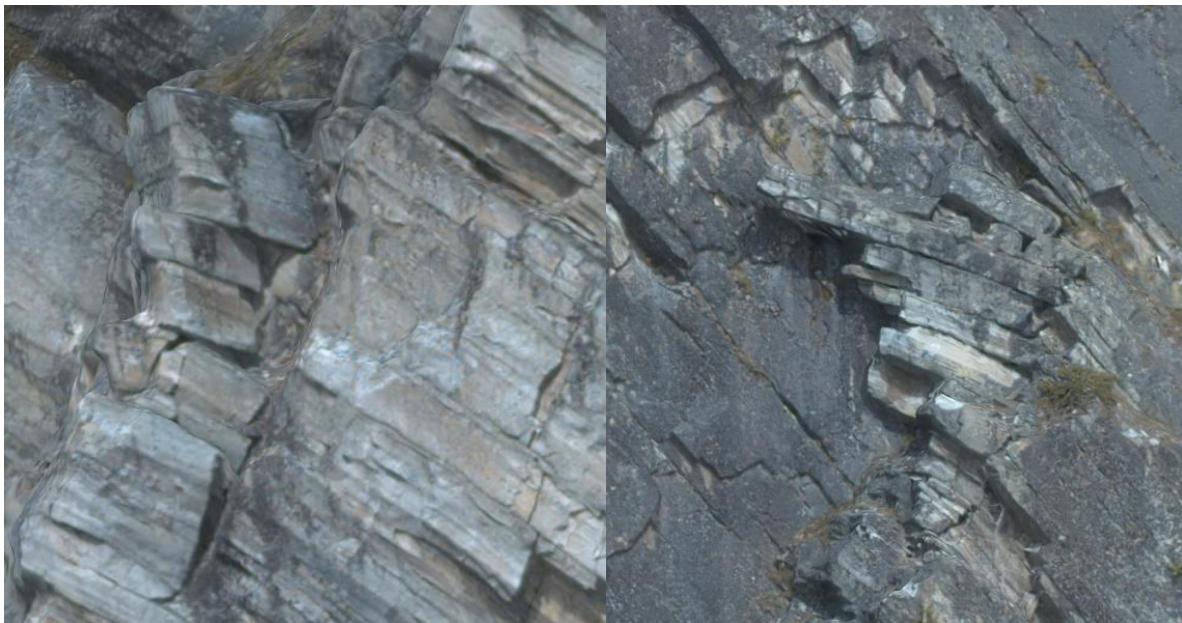
Figure 5.16 Examples of toppling blocks in Tunhovd study area, shown on the 3D mesh model. While the situation in the left figure resembles direct toppling, the situation in the right figure looks more like flexural toppling.
