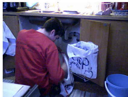
Figure 7.8: P-observe fixes a faucet in the kitchen.
