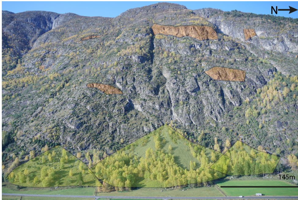
Figure 3.3: Overview picture of a typical area with a talus slope and steep rock wall with multiple potential rockfall source areas in Lærdalen. Some of the most apparent unstable rockfall source areas showing potential loose blocks are marked in orange. Three talus slopes are marked in green. Photo by: Lin Alexandra Emhjellen.
