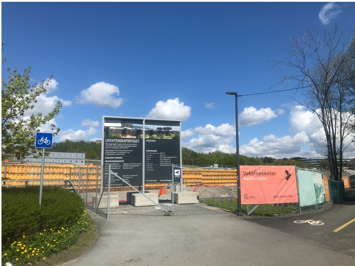
Figure 25: Photo of current situation of building LSB
