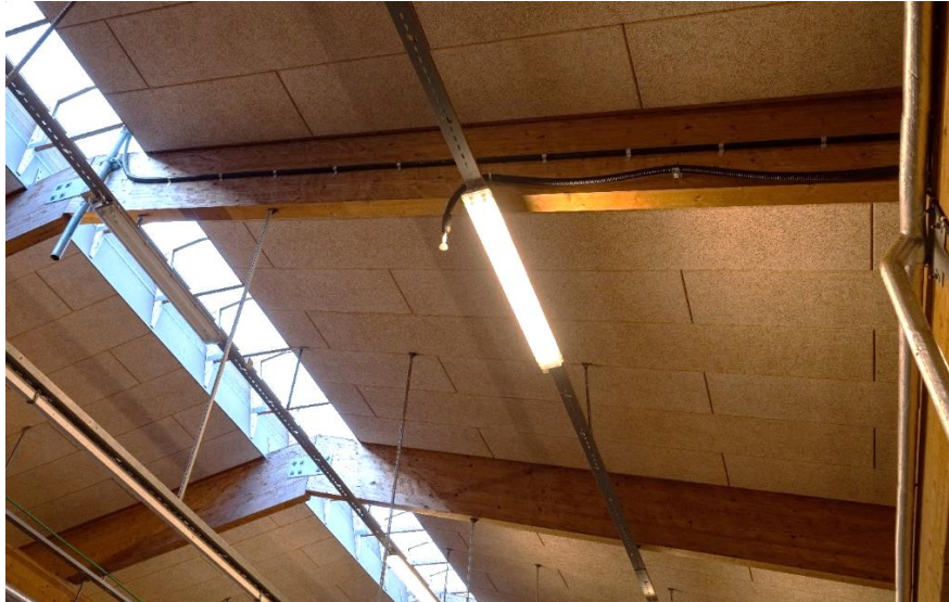
Figure 2.6: An illustration of the inlet of the heated line. The inlet was installed close to the center of the roof of the barn. The windows along the roof contribute to the natural ventilation of the barn.
