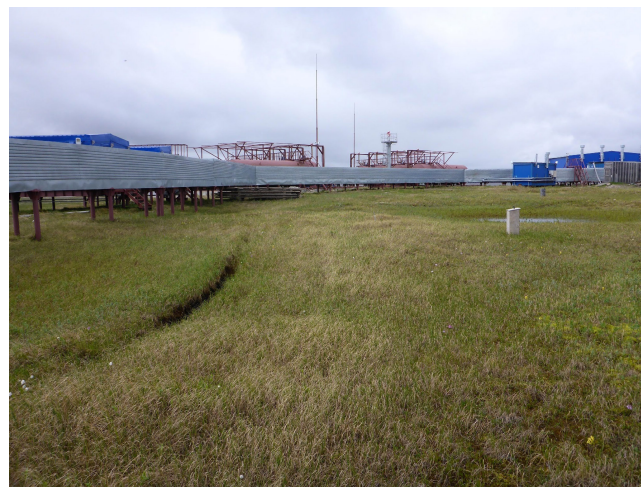
Figure E4. Borehole location (wooden box on right side) with the new Samoylov research station and water supply system (silver metal structure extending above the tundra surface).
