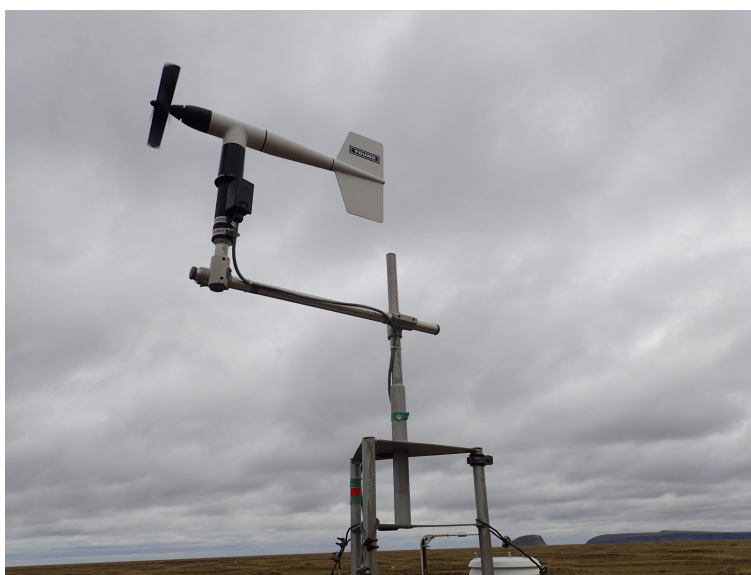
Figure B2. Young 05103 wind monitor for measuring wind direction and speed, installed on 31 August 2002.
