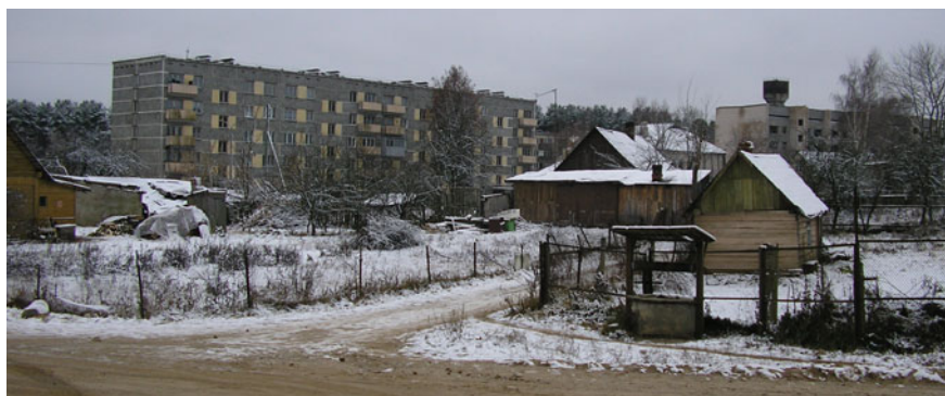
Fig. 3.5 Križi, an unfinished and isolated mikrorajon in Daugavpils. A well for the residents of the single-family housing is visible in the foreground. Source Michael Gentile
