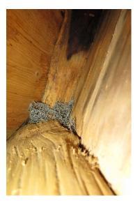
Figure 59. A method for preventing bats to re-enter the building is to seal bat entry holes.
