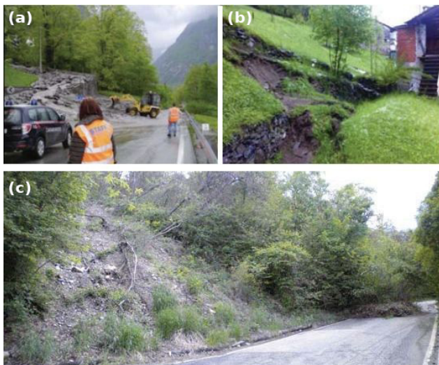
Figure 15. Some examples of slope phenomena recorded during rainfall event. (a) Road interrupted by a debris flow; (b) a building hit by small rotational slide; (c) shallow landslides on a road (source: Regione Piemonte).
