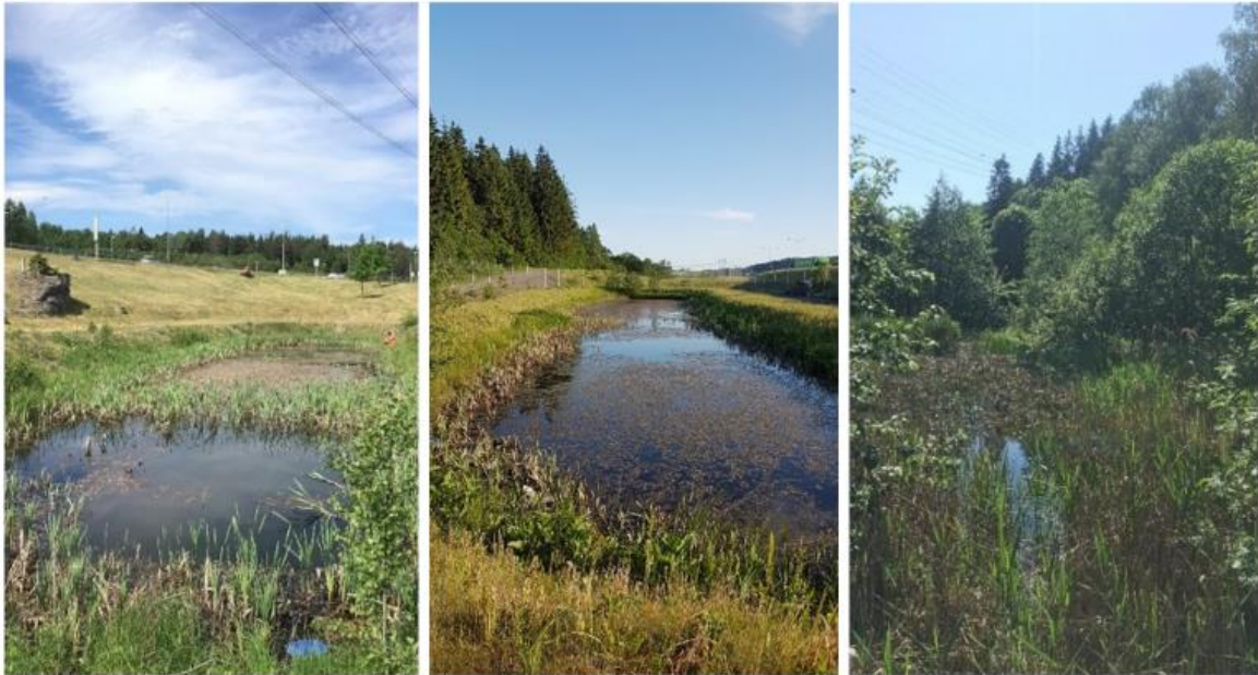
A8 – Taraldrud South, Tveiten and Vassum sedimentation pond
