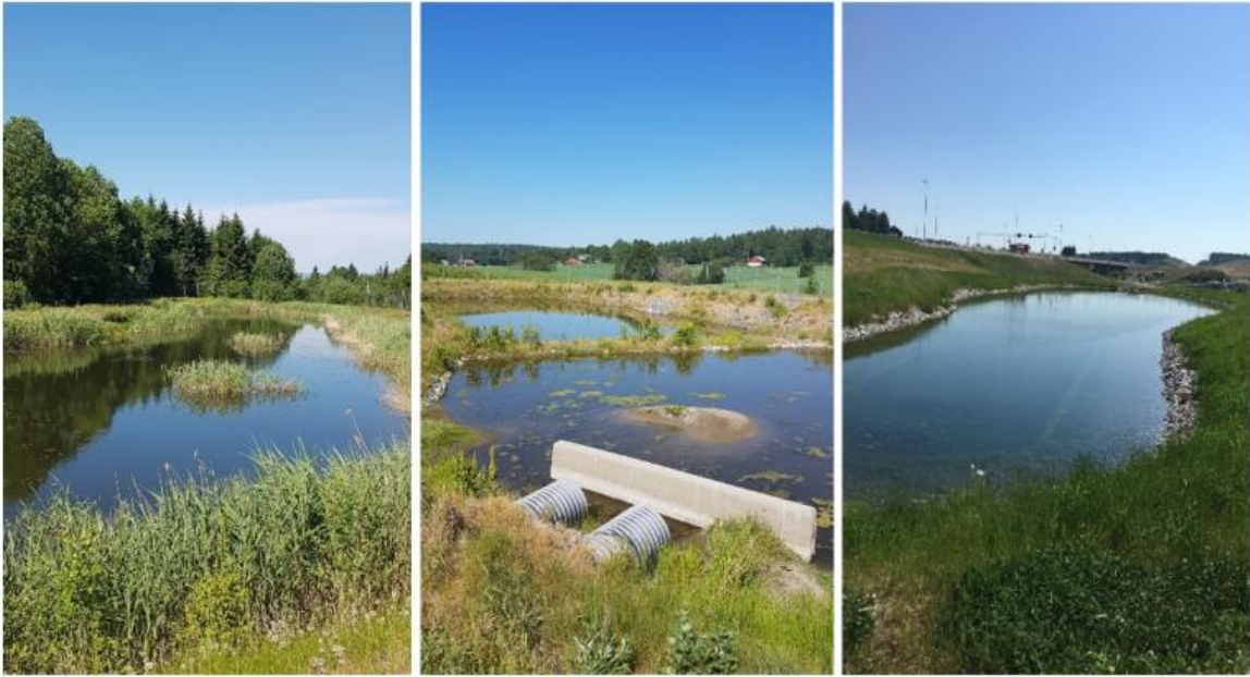
A3 – Helland, Holmane and Holt sedimentation pond
