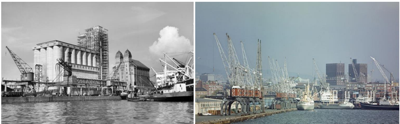
Figure 2.6 Images from the industrialized history of Oslo harbor including the grain silo at Vippetangen (left) from Wilse (1935) and the Oslo harbor area near Filipstadkaia (right) circa 1970 (Ørsted, 1970).
