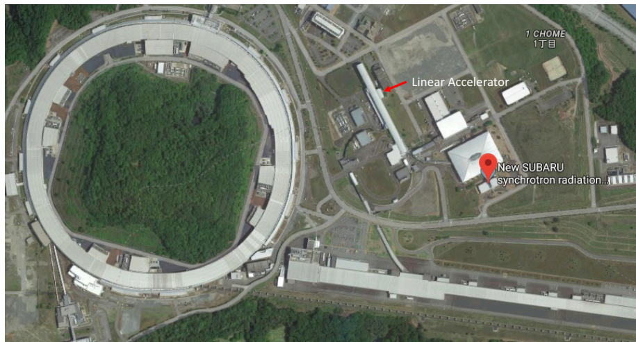
Figure 4.1: View of the SPring-8 accelerator complex. The complex is composed of a 1 GeV linac, 8 GeV booster synchrotron, 1 GeV NewSUBARU storage ring and 8 GeV SPring-8 storage ring. Figure taken from [74].
