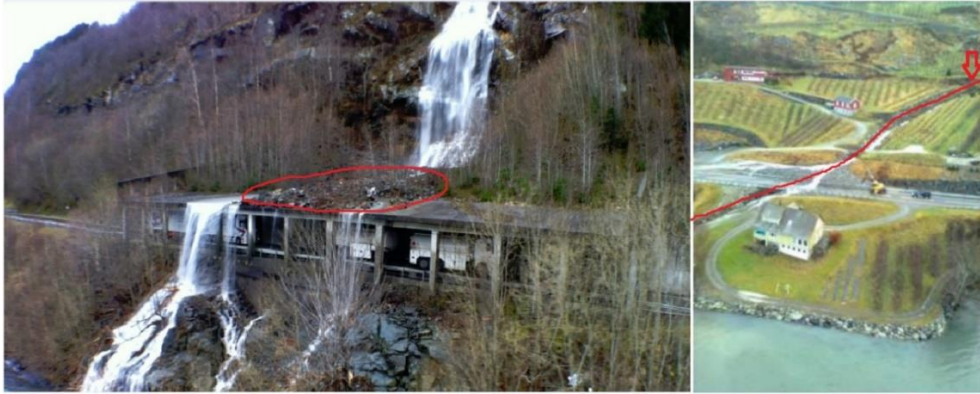
Figure 5.11: Examples of the use of photographs. Left: Picture of a landslide hitting a mitigation measure along Sør fjorden. The news coverage focused on the trailers trapped below it, as the road on both sides was blocked by other landslides, but this landslide was not registered in the database. Deposit material is shown with a red circle (Source; NRK). Right: Example of a landslide that might have the wrong date in the database, because of contradicting sources. The picture shows a debris flow after “Dagmar” 2011 from the NPRA, with the red line showing where the track is.
