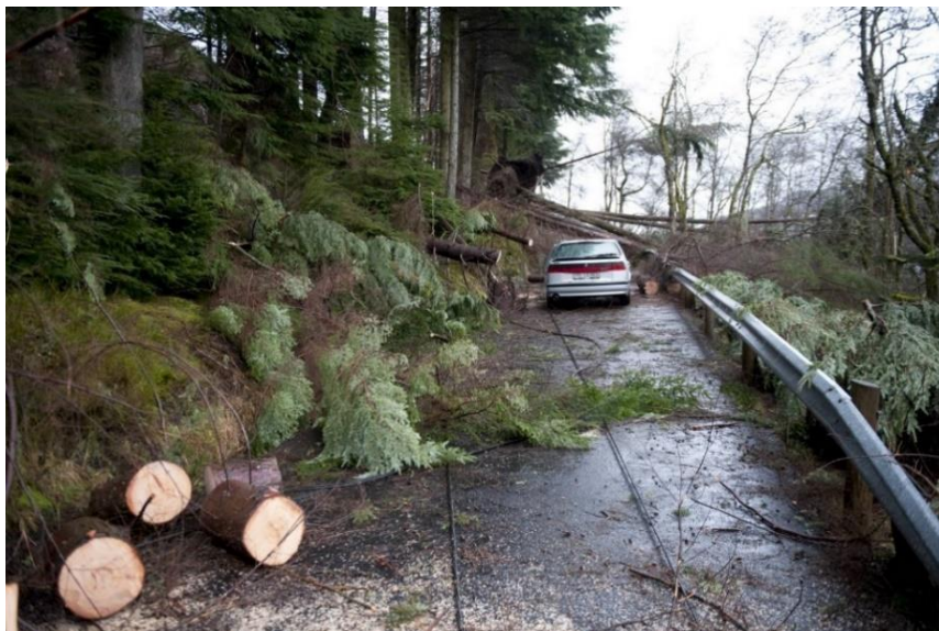
Figure 7.3: Cleanup of fallen trees in Kismulvegen in Bergen after “Berit” (2011). Other trees were also cut as a preventive measure to avoid similar damages at future storms. (Source: Bergensavisen/Arne Ristesund)
