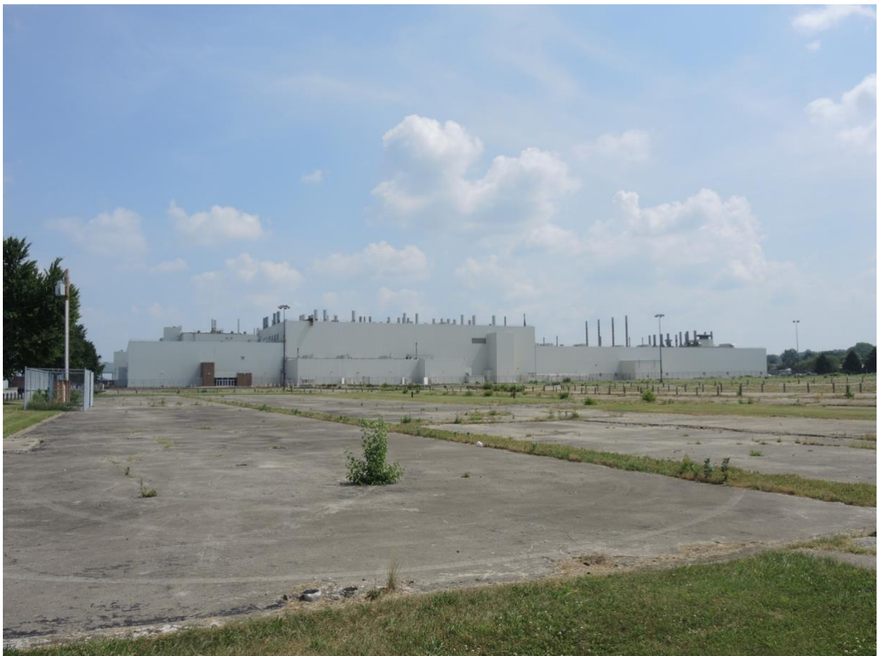
Figure 6 A part of the Moraine plant complex not in use. Picture taken by author
