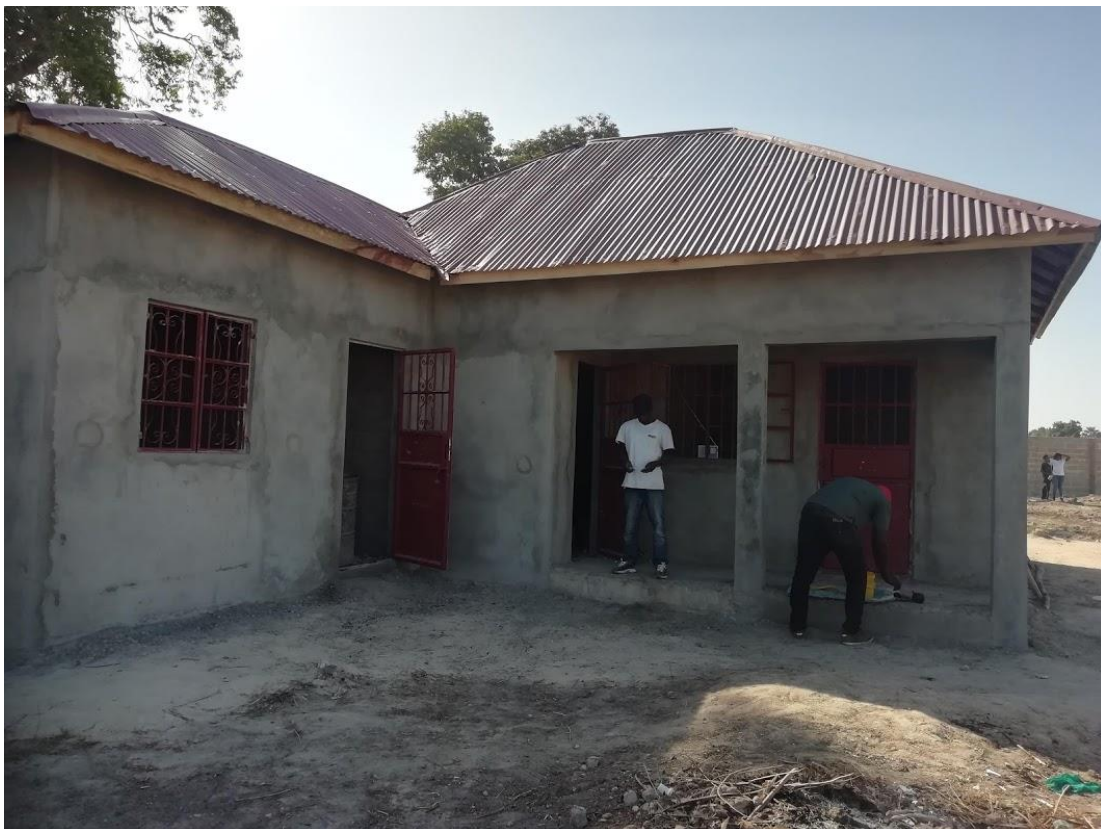
Figure 7: The Wellness Centre; the kitchen mid-build. November 2018
