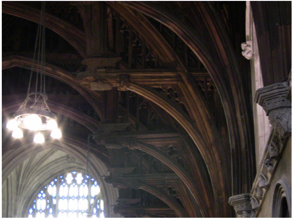
Detail from the hammer-beam roof of Westminster Hall, the oldest building on the Parliamentary Estate. Parliamentary copyright images are reproduced with the permission of Parliament.
