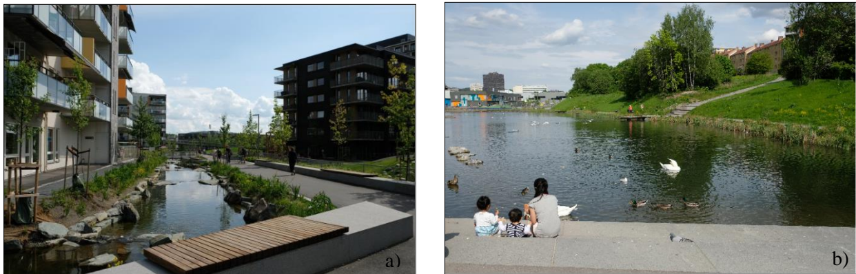
Figure 3.5: a) Daylighting of Hovinbekken and b) Teglewerksdammen. Photos from Gulde (2017).
