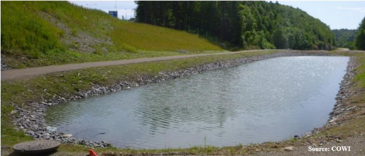
Figure 6 - Sketch of a wet sedimentation pond, and a recently built pond.
