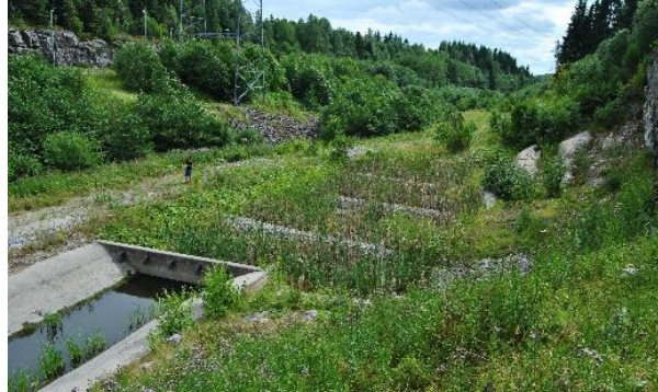
Figure 8 - Nøstvedt sedimentation pond. Source: NPRA
