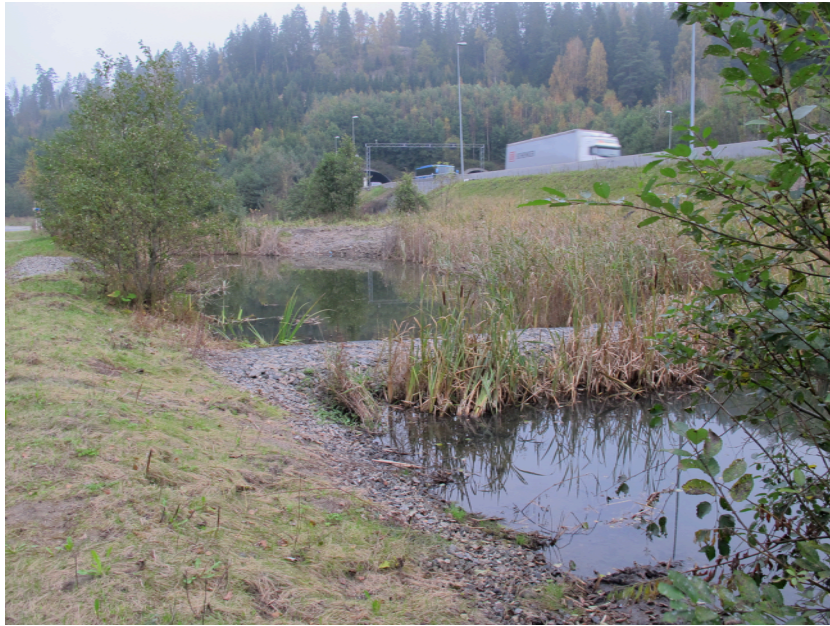
Figure 2.1.1: Vassum sedimentation pond with Norbyttunnelen in the background. The pre-sedimentation pond is seen in front and the main pond in the back. Photo: Kjersti Wike Kronvall
