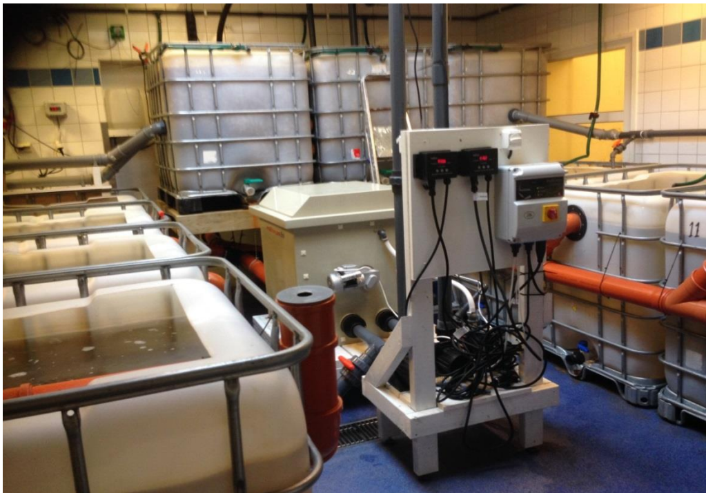
Figure 9 The fish feces are pumped into the highest tank where the ammonium is converted into nitrate.
