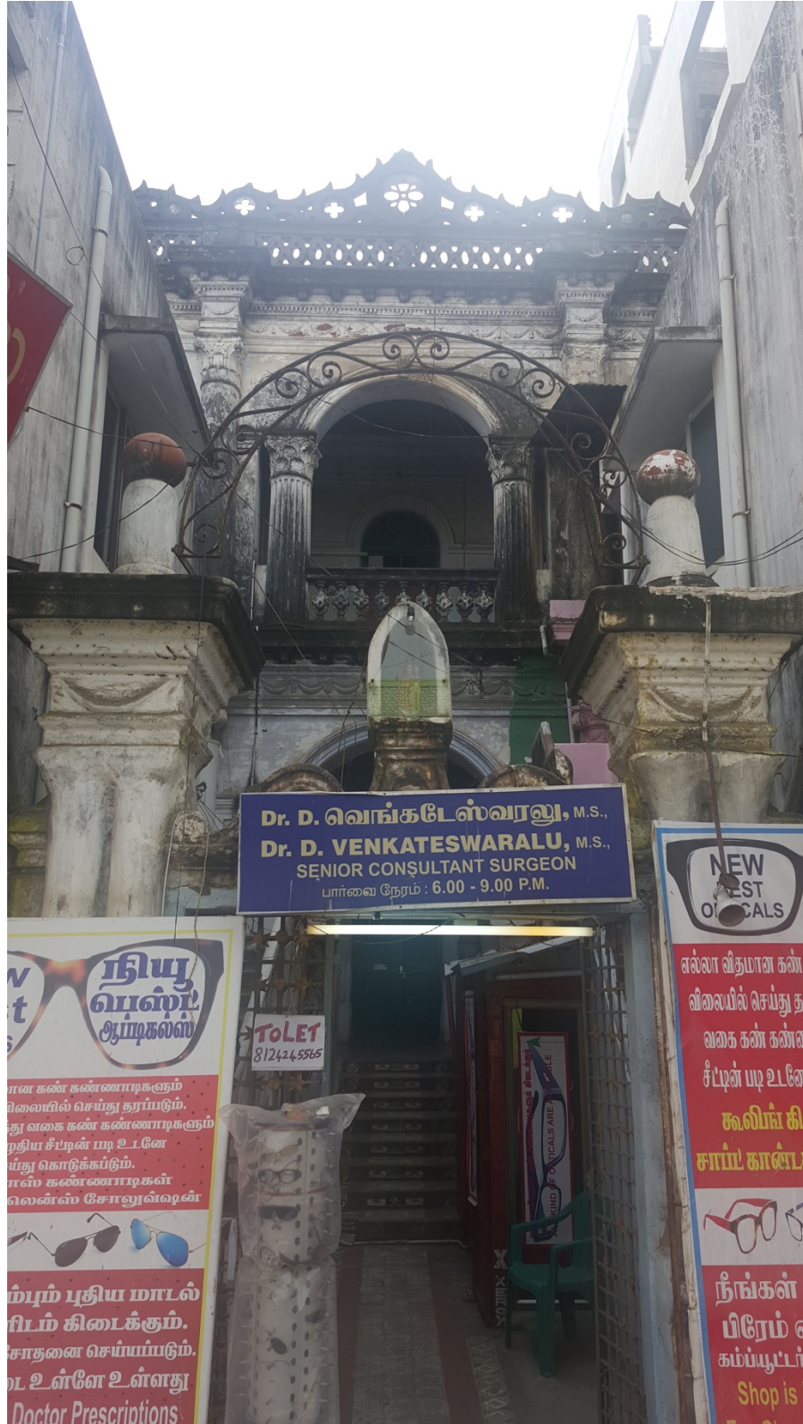
Fig: 7 An example of a decaying heritage building. Photo by Author
