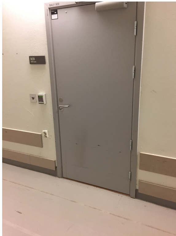
Figure 6.11: Conflicting door with the path of the AGV
