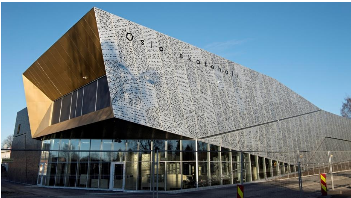
Figure 51 Oslo Skatehall façade
