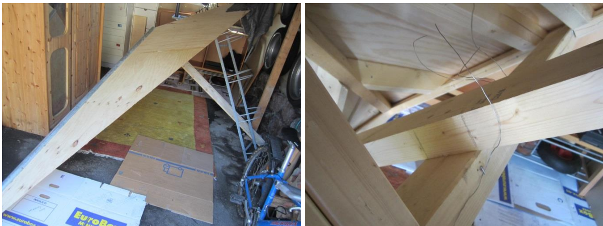
Figure 44 Wiring the prototype
