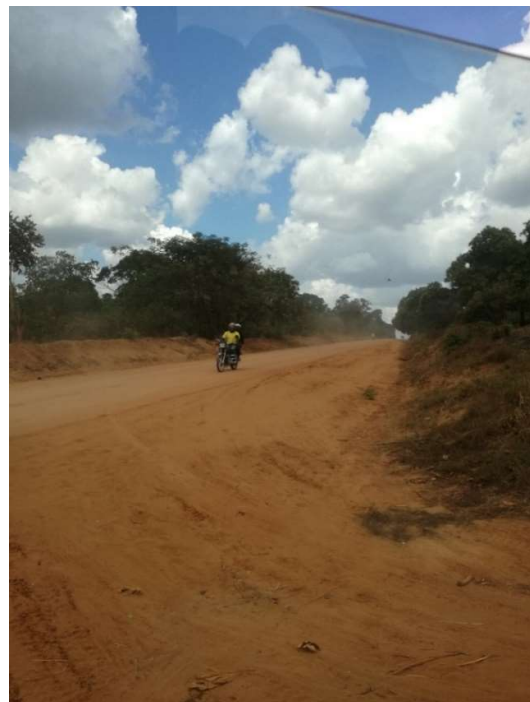
Figure 7 - Example of the road quality in a rural area
