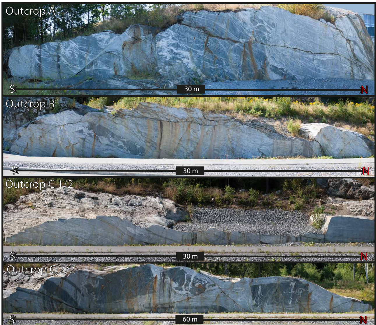
Figure 1.1: The outcrops (A, B & C) investigated in this study, located at Remmen, Halden (Østfold).
