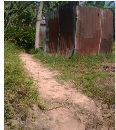
one of the sanitary facilities at Rukiga Primary school.
