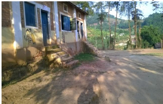
some of the class rooms with stairs at Nyakigugwe primary school
