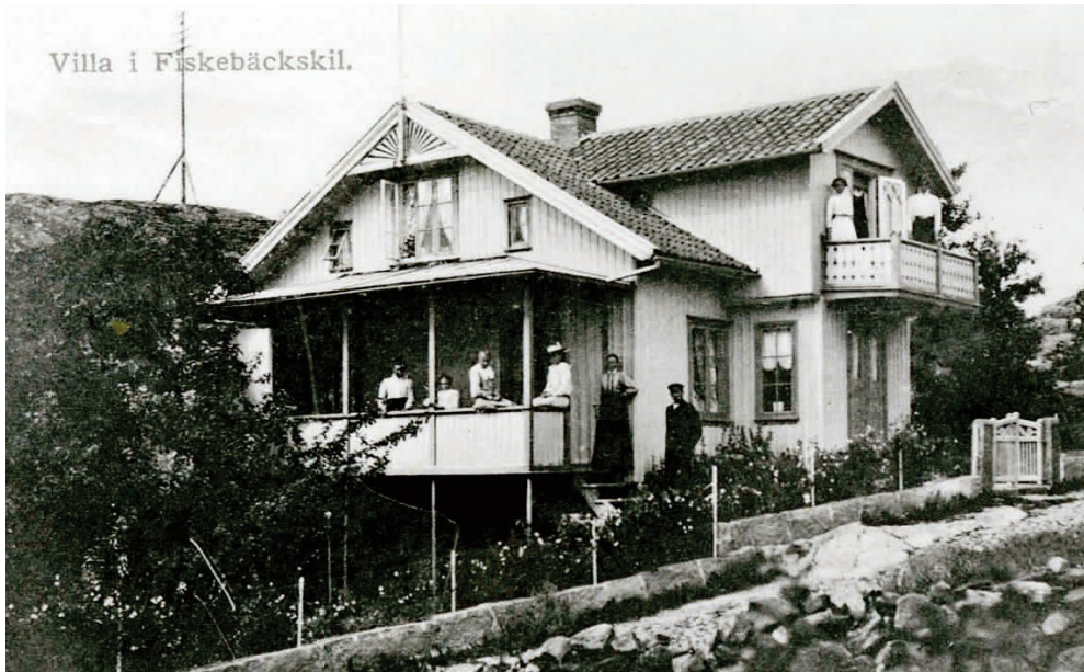
A boarding house in Fiskebäckskil at the beginning of the twentieth century. At that time many better-off families, particularly among the shipmaster population, had houses built that were larger than they needed for their own use. They built the houses with the intention of renting them out, as was the case with this big house. Photo Gothenburg Historic Museum.
