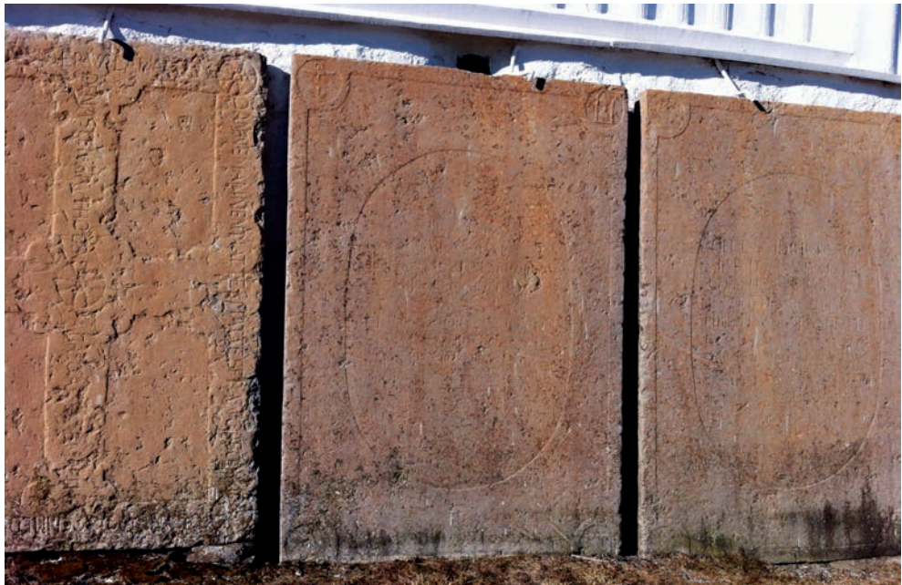
44. Three grave slabs that were moved from the church floor in Fiskebäckskil and raised along the outer church wall. The original text has been worn out and is for the most part illegible due to the earlier pressure of walking feet while the stones lay on the church floor.
