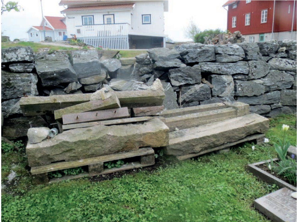
52. Granite frames in Käringön that have been removed and placed near the cemetery wall. The alternative is to crush them.
