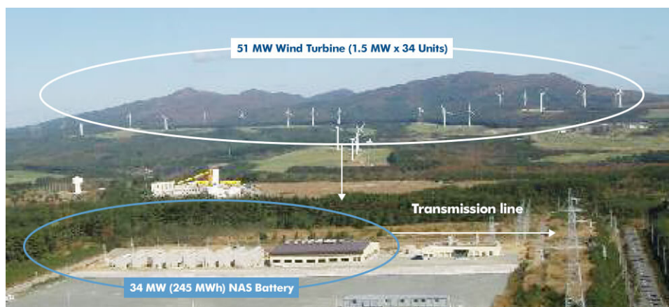
Figure 1.1: Wind farm and NAS batteries installed in Rokkasho (Japan) [4]
