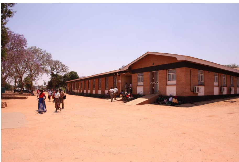
Figure 3.3 – A health facility in Malawi
