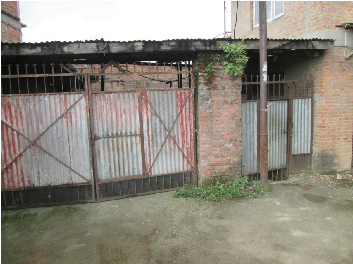
Figure 5: The entrance to a factory (photo: author)
