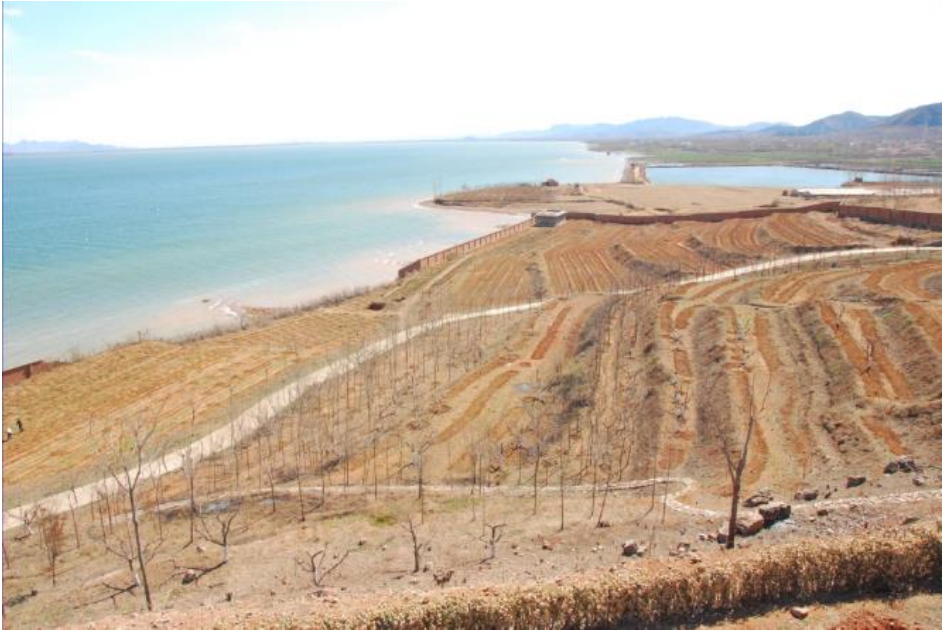
Figure 19 Terraced farmland in the south shore constructed to reduce runoff and erosion. (Photo: Dr. Xueqiang Lu).
