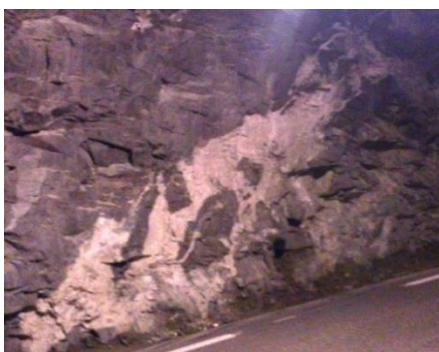
Figure 95 - Quartz vein cutting eclogite in the tunnel. Vein contains several larger rutile crystals.
