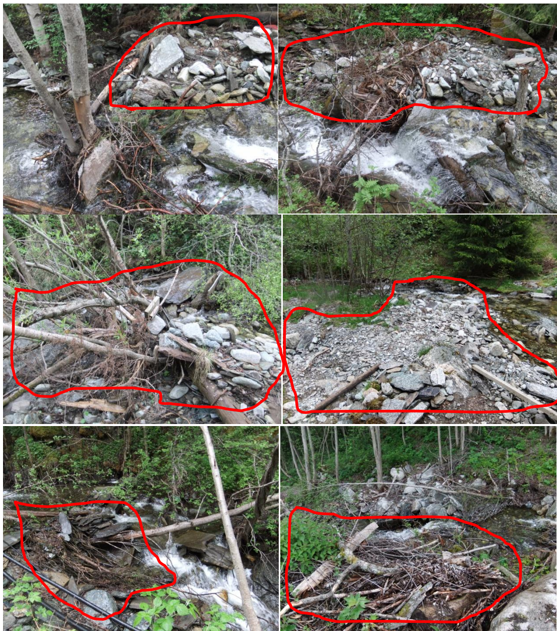
Figure 5.3.2 Debris deposit along the track.
