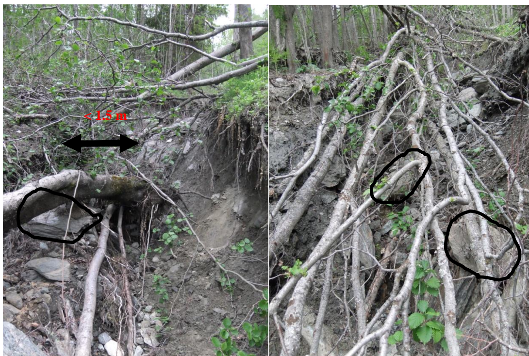
Figure 5.2.2.5 Woods dams in point 132 (left) and point 128 (right).
