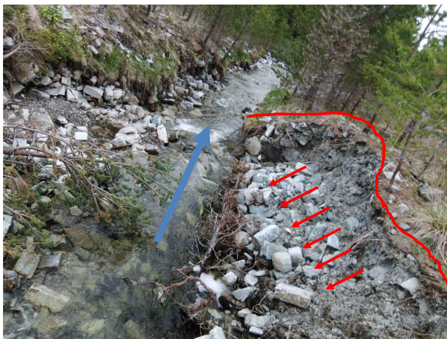
Figure 5.3.2.5 The failure slope in the end of the dumped waste, the blue arrow showed the flow direction.
