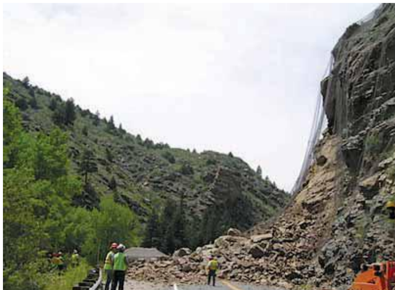
Figure 3.2.1 A rockfall occurred in Colorado Usa in 2005, photograph by Colorado Geological Survey (Highland 2008).
