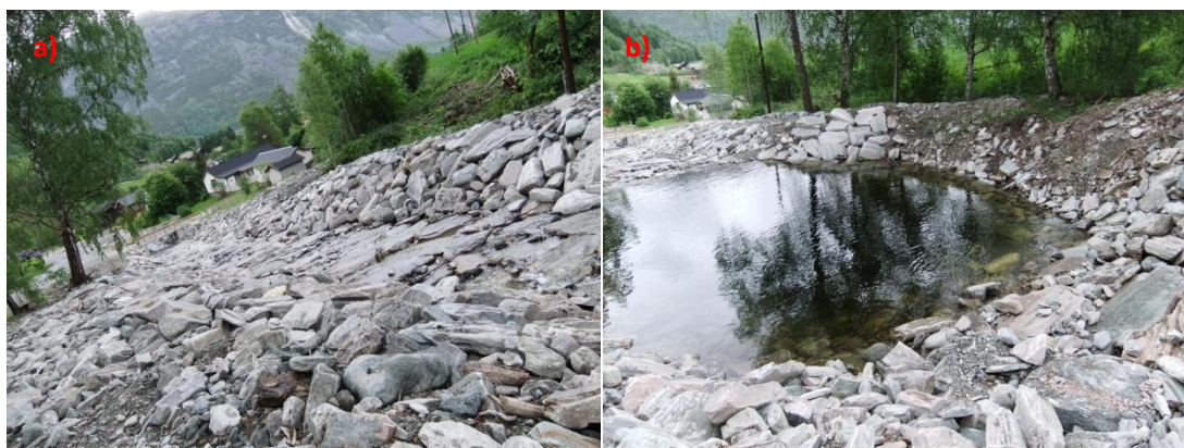
Figure 5.3.2 a) the readjusted channel, b) the built pool for risk mitigation.
