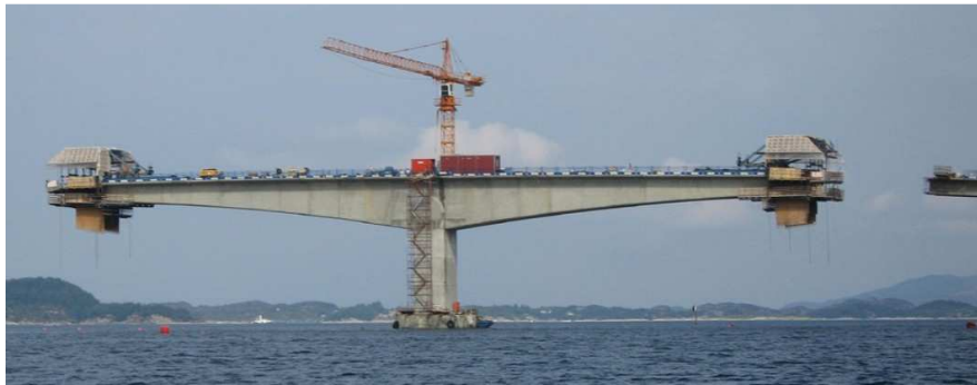
Figure 33 – A concrete cantilever bridge during construction
