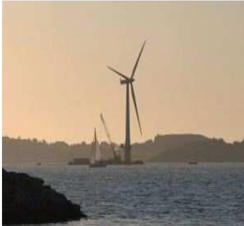
Figure 1: Hywind turbine installed in the North Sea, Norway in 2010. Image source http://en.wikipedia.org/wiki/File:Hywind.jpg
