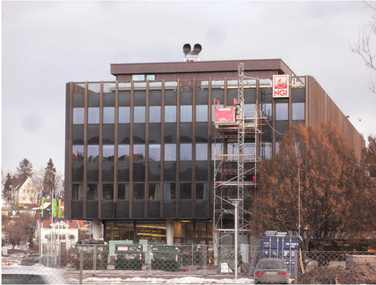
Figure 10.1.1: The radar on the roof of the building.
