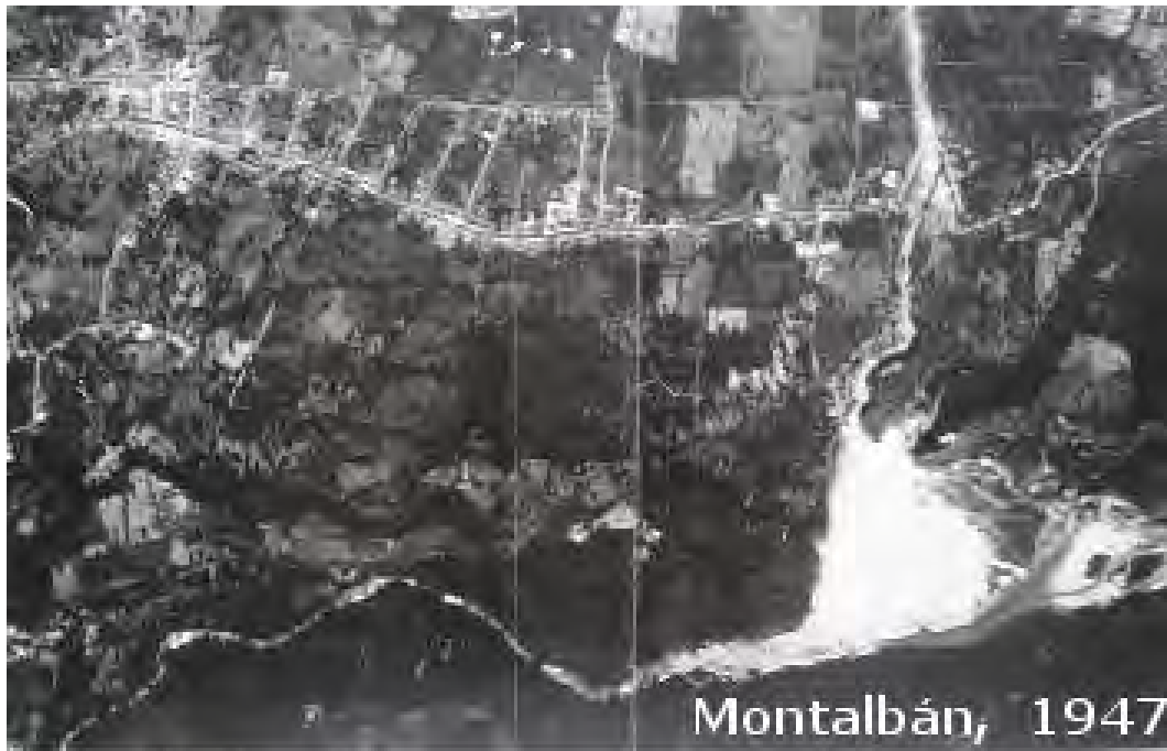
Figure 6.8: MONTALBÁN DEBRIS FLOW EVENT
