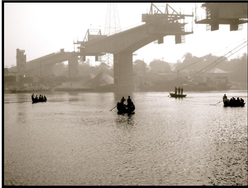
Image 12.1 Building a new bridge just outside of Dhaka City
