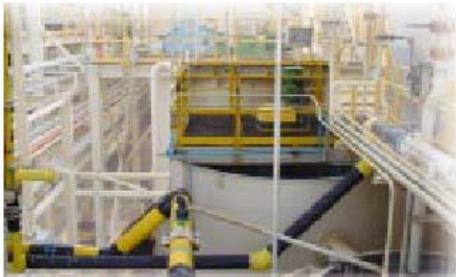
Picture2) The INCO circuit that destroys free and weak acid dissociable cyanide.
